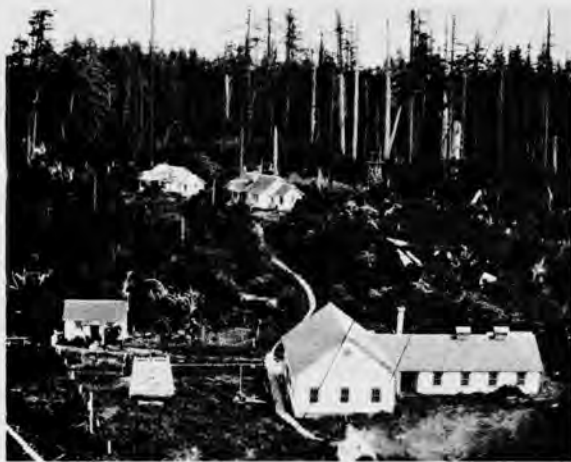
Small shed in foreground was distillery for battery water. Large building also in foreground, contained workshop, engine room, and battery room with 120 volts to run transmitters. To the left was the cooler for the 50 h.p. semi-diesel, behind this was the truck drivers house. The first house in the background was the O.I.C.'s, the second an operators. To the right of these houses was the water storage tank with a well underneath. . . water was very harsh, with a high content of iron. (Courtesy N. Smith)
